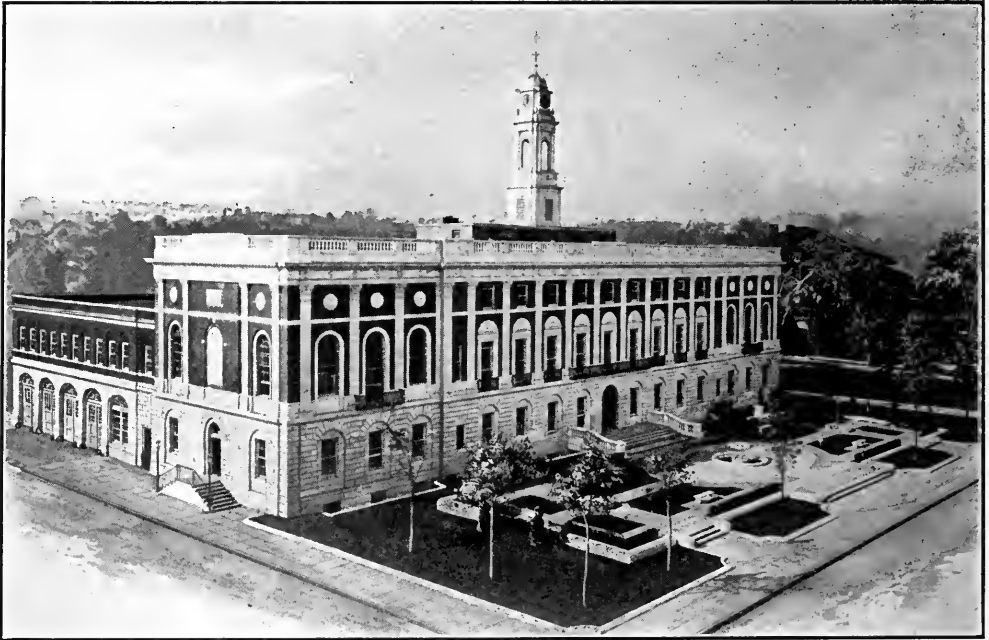
GENERAL VIEW OF THE WATERBURY, CONN., CITY HALL
